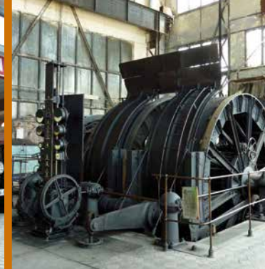
Michal Mine, Ostrava, Czech Republic
