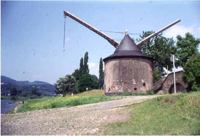
A crane for loading barrels of wine on to barges alongside the River Mosel at Trier.
