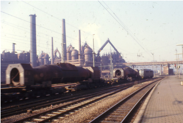
A distant view in 1989 of the blast furnaces at Volklingen in the Saarland, before the commencement of large-scale restoration work. The train in the foreground had delivered liquid steel in torpedo wagons to a nearby steelworks.
