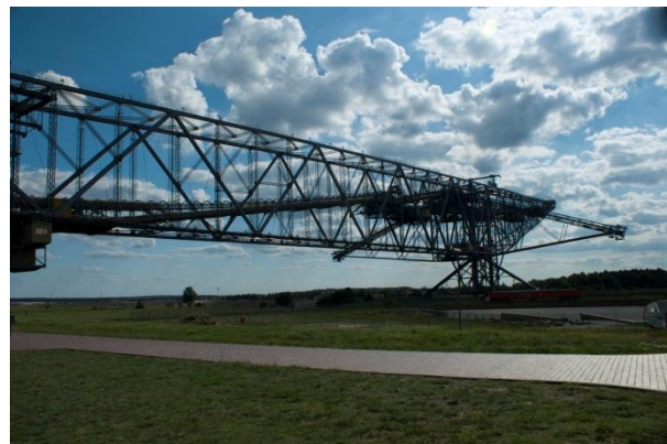
Conveyor bridge F60 in Lichterfelde. Julia Petzak.
