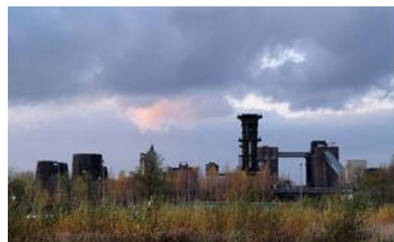
Facilities of the coking plant Hansa in Dortmund. Arnoldius.
